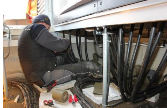
Assembly conditions in the solar park
