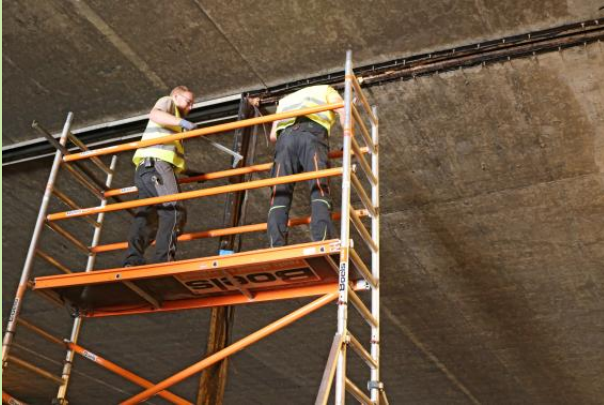
Inspection of the ceiling joint cavities during the tunnel closure period
