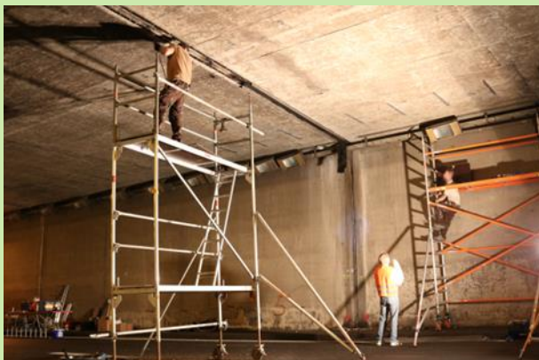
Construction crews 3 and 4, Stuttgart direction
