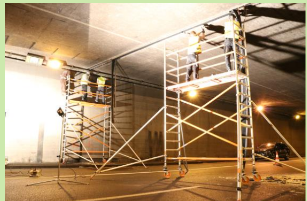
Construction crews 1 and 2, Singen direction
