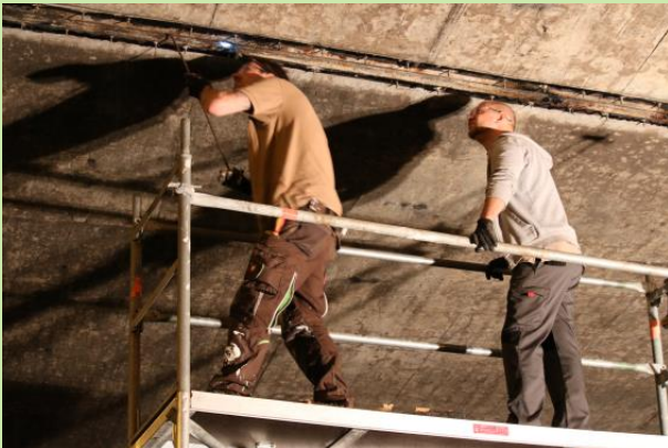
Inspection of the ceiling joint cavities during the tunnel closure period
