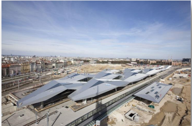
Main station, Vienna, Austria Source: Architekten24 Photo © Unger Steel Group, Renée Del Missier
