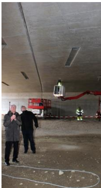
Photo left: All previous sealing material was removed from the expansion joint up to a depth of 80 cm
