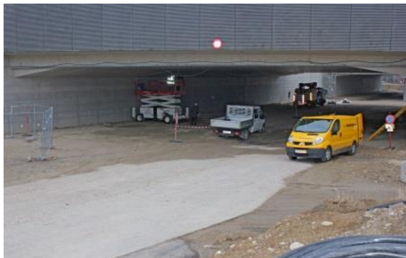
Photo right: Mobile working platform
