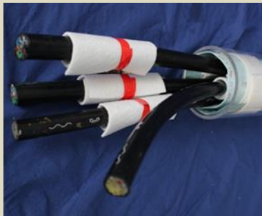
Reinstall the sealing cushion
