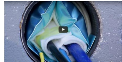
Installation/ removal cable protection duct seal Ø ≥ 80 mm
